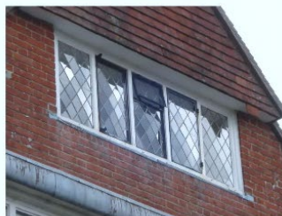
External window - dormitory room 10
