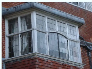
External window - dormitory room 3
