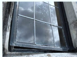
Detail of leaded lights (external) - Main Hall
